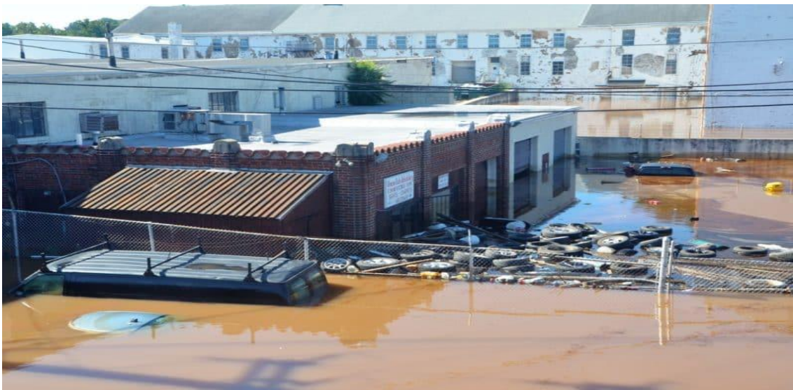
Flooding in Norristown, PA from remains of Hurricane Ida (September 2, 2021).
