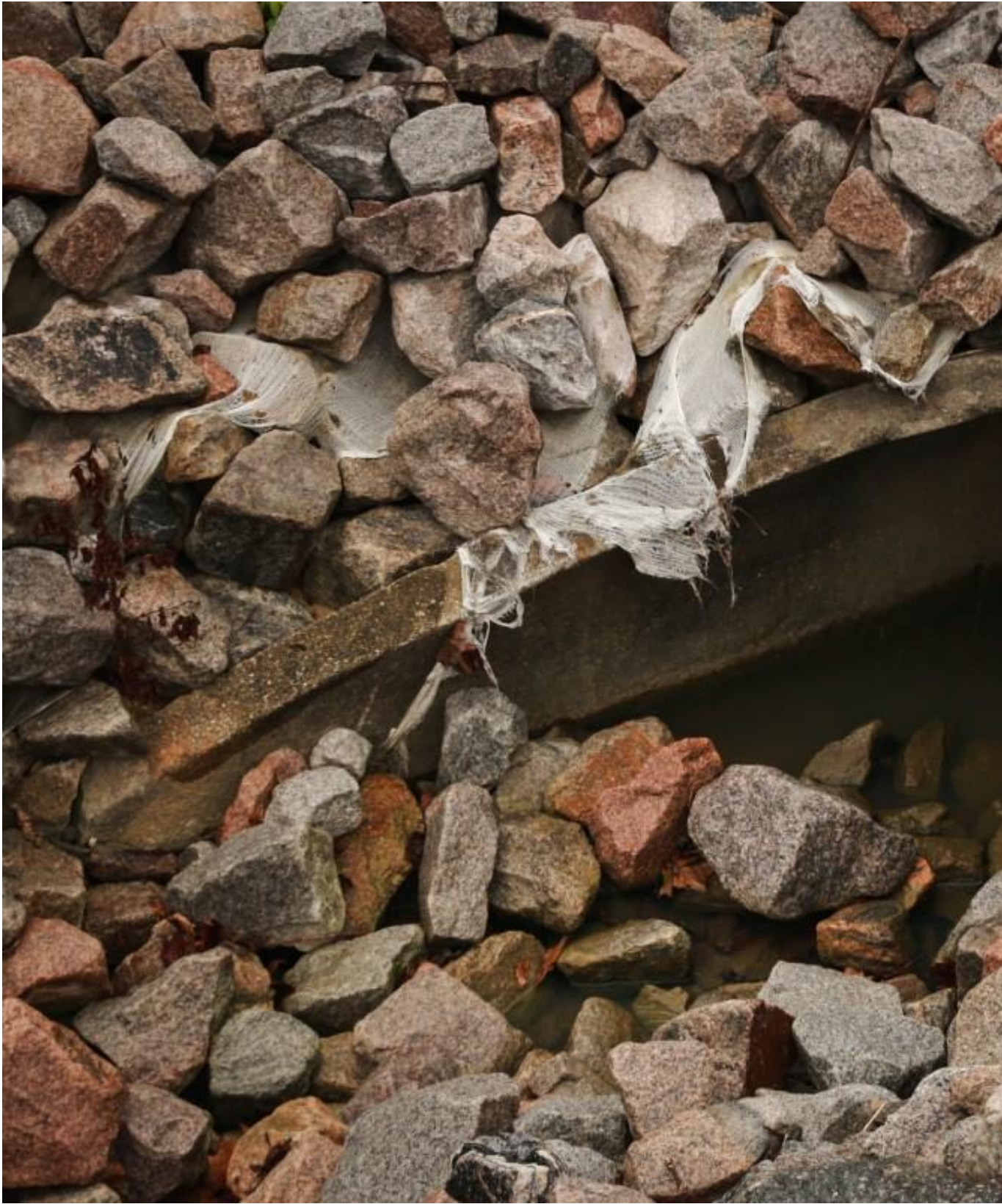
Stormwater outfall and riprap in front of Braven's facility on Sep. 17, 2023.
